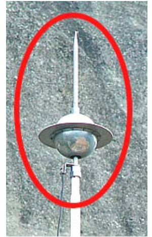
(B) "ESE" (Early Streamer Emission) (a theorized "ion-path generator", to ATTRACT a hit)
