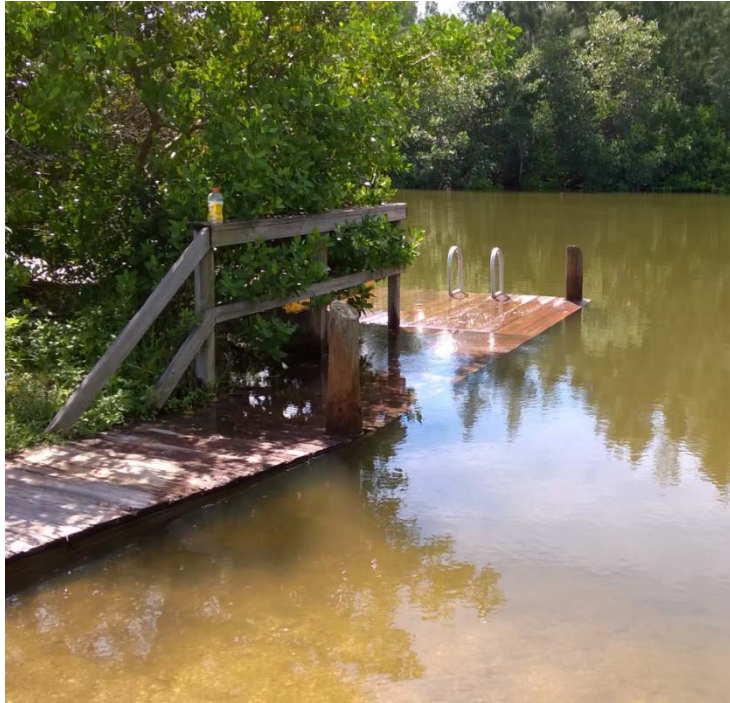
Ramp Road, City Dock
