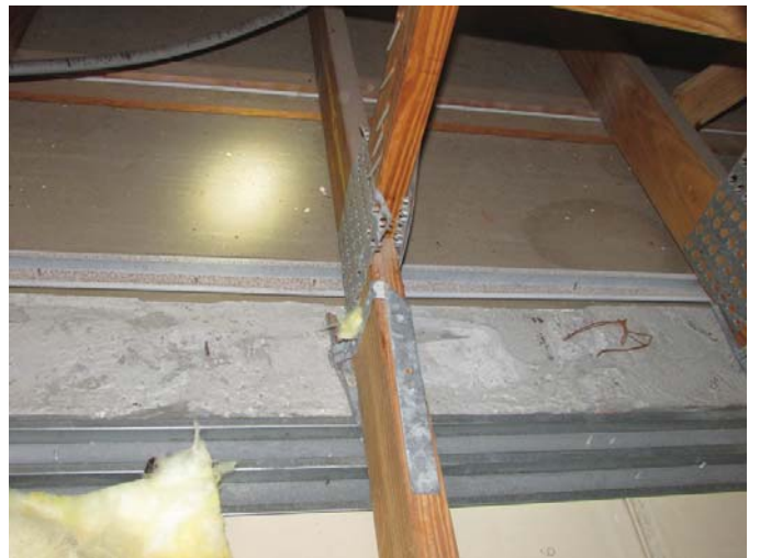
Clip with a minimum of 3 nails (opposite side)
