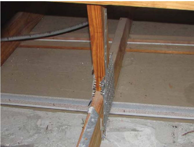
Clip with a minimum of 3 nails
