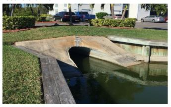
The repair work encompasses demolition of the concrete above the waterline, grading the area with stone, place commercial fabric at the bottom and edges of area to be formed and poured, and place wire mesh. Form and pour 6 inches of concrete and remove the forms, completing the job. During this repair, the roadway on the south side of Building 4 garage may be closed while the main thoroughfare will not be closed.
